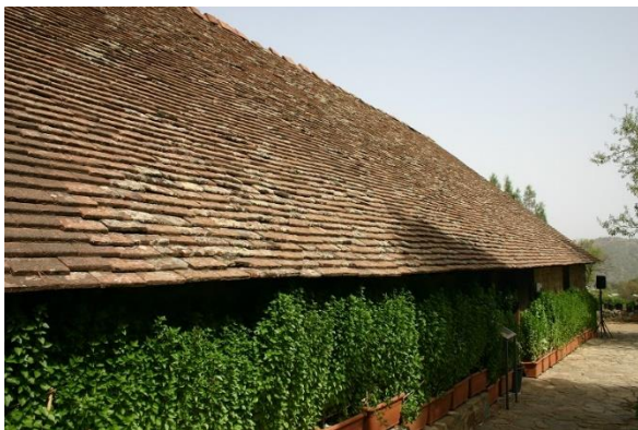
fig. 4.6 The tiles on the roof of the church at Platanistasa
