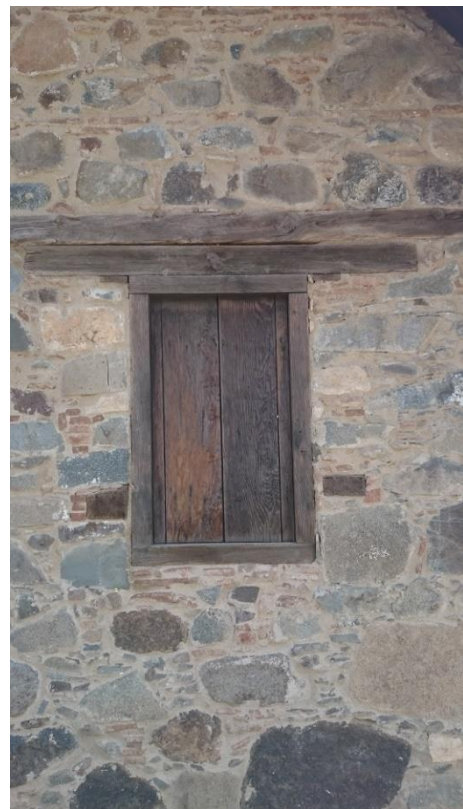
fig. 5.8 Windows were in most cases a later addition and were placed on the long side of the church when there were not any door. The size is very small and the lintel here is the wall plate
