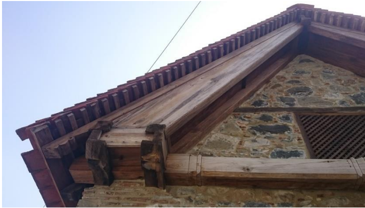
fig. 3.4 Details showing the four wall plates
