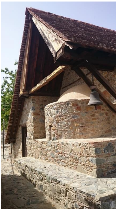
fig. 5.10 The dome of the church in Pedoulas. A part of it is covered by the roof.
