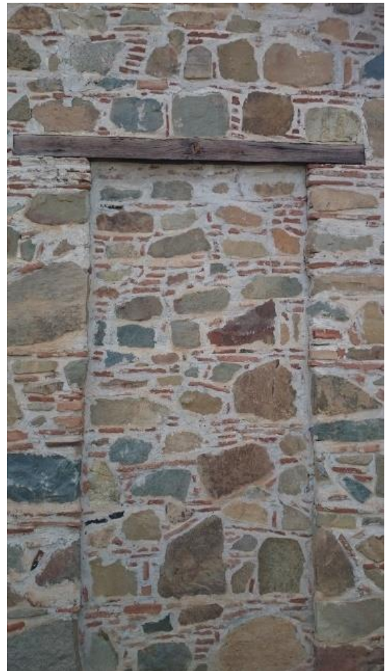
fig. 5.6 A photo of the masonry showing clearly the materials, the colours and the textures. In this case, it looks like there was one door opening being covered later with masonry
