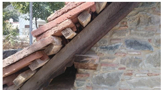
fig. 4.4 Detail showing the purlins supporting the tiles
