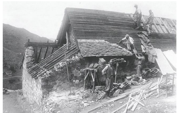
fig. 3.2 Church of the Virgin of Moutoullas during construction
