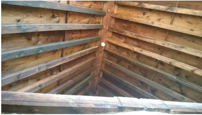
fig. 3.7 Dense position of the rafters in the internal roof construction
